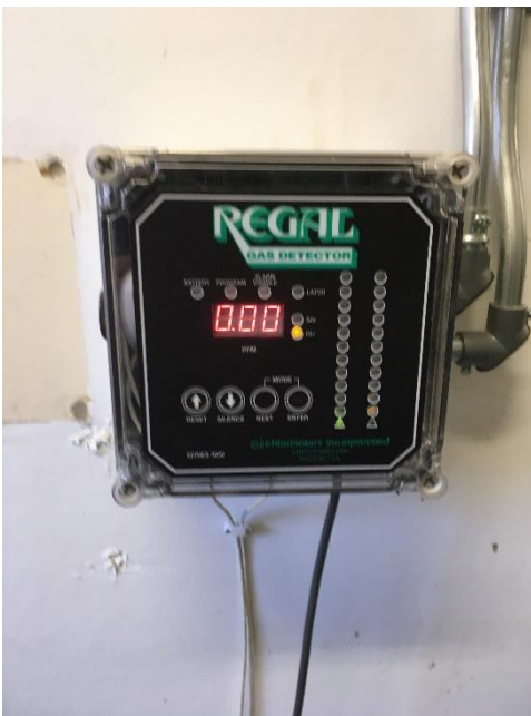
Chlorine Gas Detector
