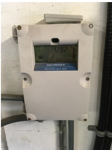
Figure 9 Ultrasonic Level Indicator
