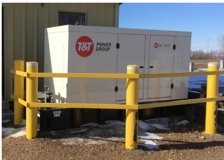
Figure 10 Standby Generator
