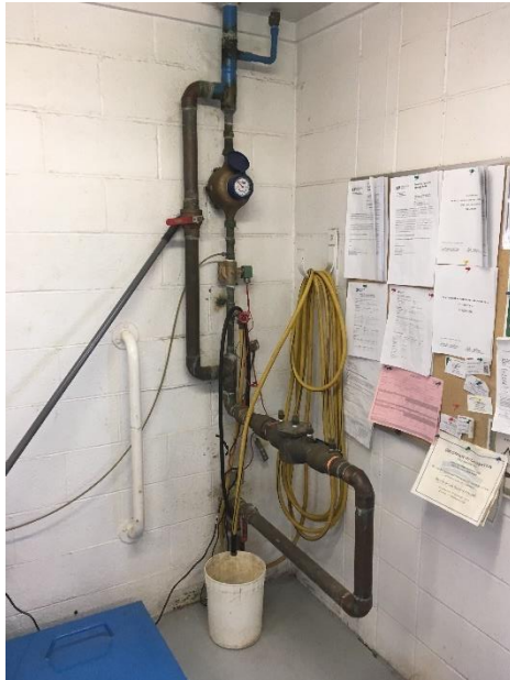
Figure 8 Backflow Prevention Device at Truck Fill Station
