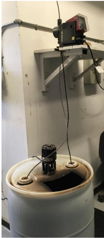
Figure 4 Potassium Permanganate Injection System
