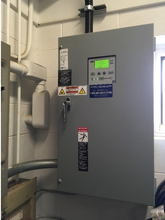
Figure 11 Automatic Transfer Switch
