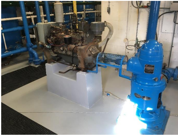
Natural Gas Engine Driven Pump
