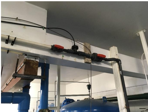
Chlorine Gas Injector
