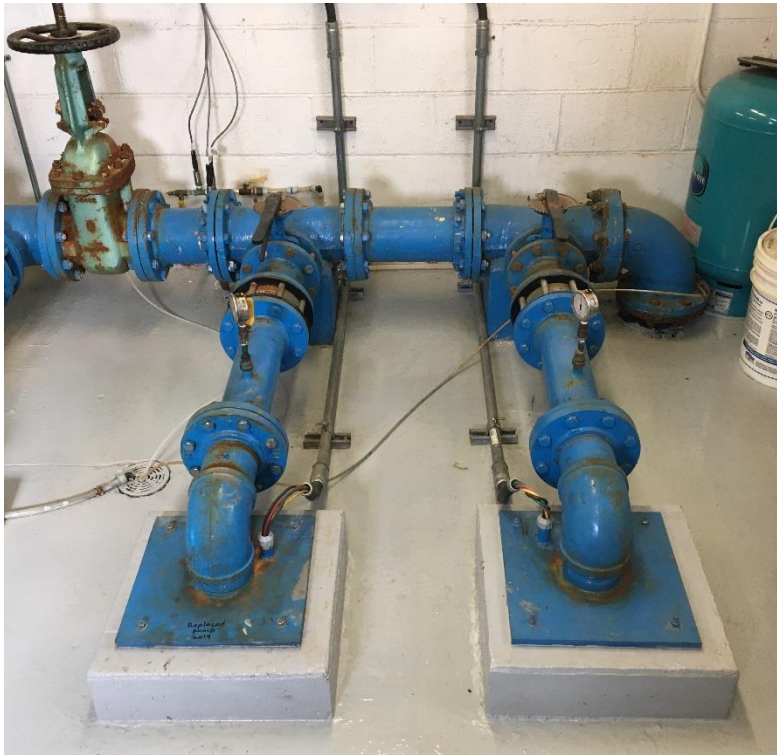
Figure 6 Submersible Distribution Pump Discharge Piping
